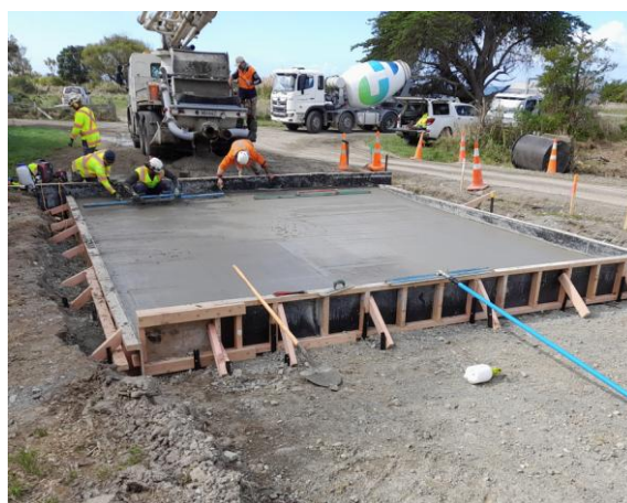
Left to right: Construction of the bund wall and concrete ford at Flat Point in the Carterton district.
